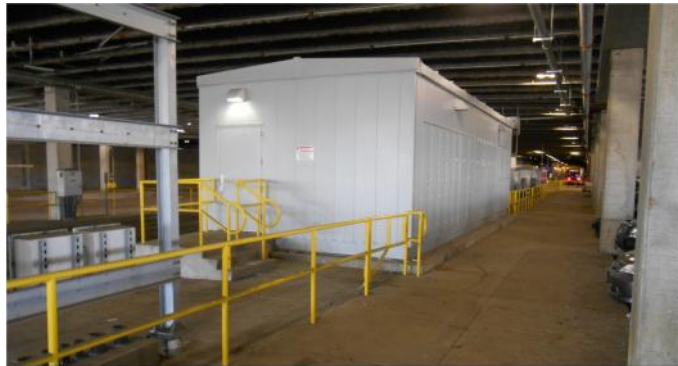
Photo 2: Build-in-Place TPSS in the Mall of America Parking Garage, Minnesota, 2014
